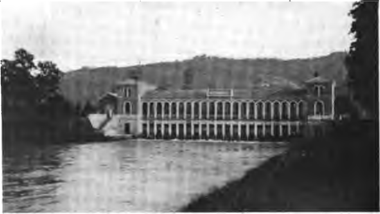
FIG. 134.—Headworks of Cavour Canal, Po River, Italy.
